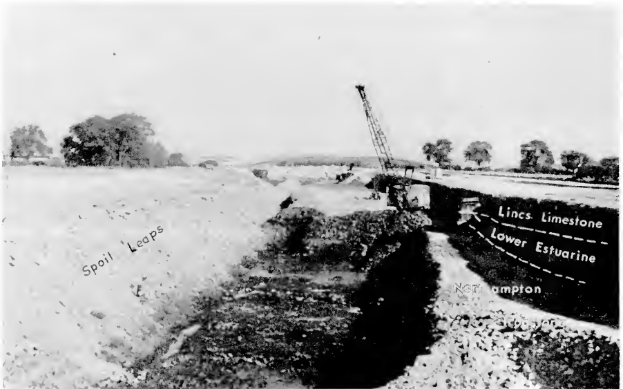
Plate 3. Stainby Glebe quarry: Northampton Ironstone overlain by Lower Estuarine and Lincolnshire Limestone. (SK 917235). (Photo by D. N. Robinson)
